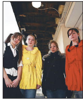
Concerns: Residents Jessie Pennings, 14, Emily Kerr, 14, Georgina Kovacs and Jodie Chard, 12, under a damaged roof
